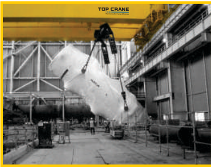
Power Plant Cranes
